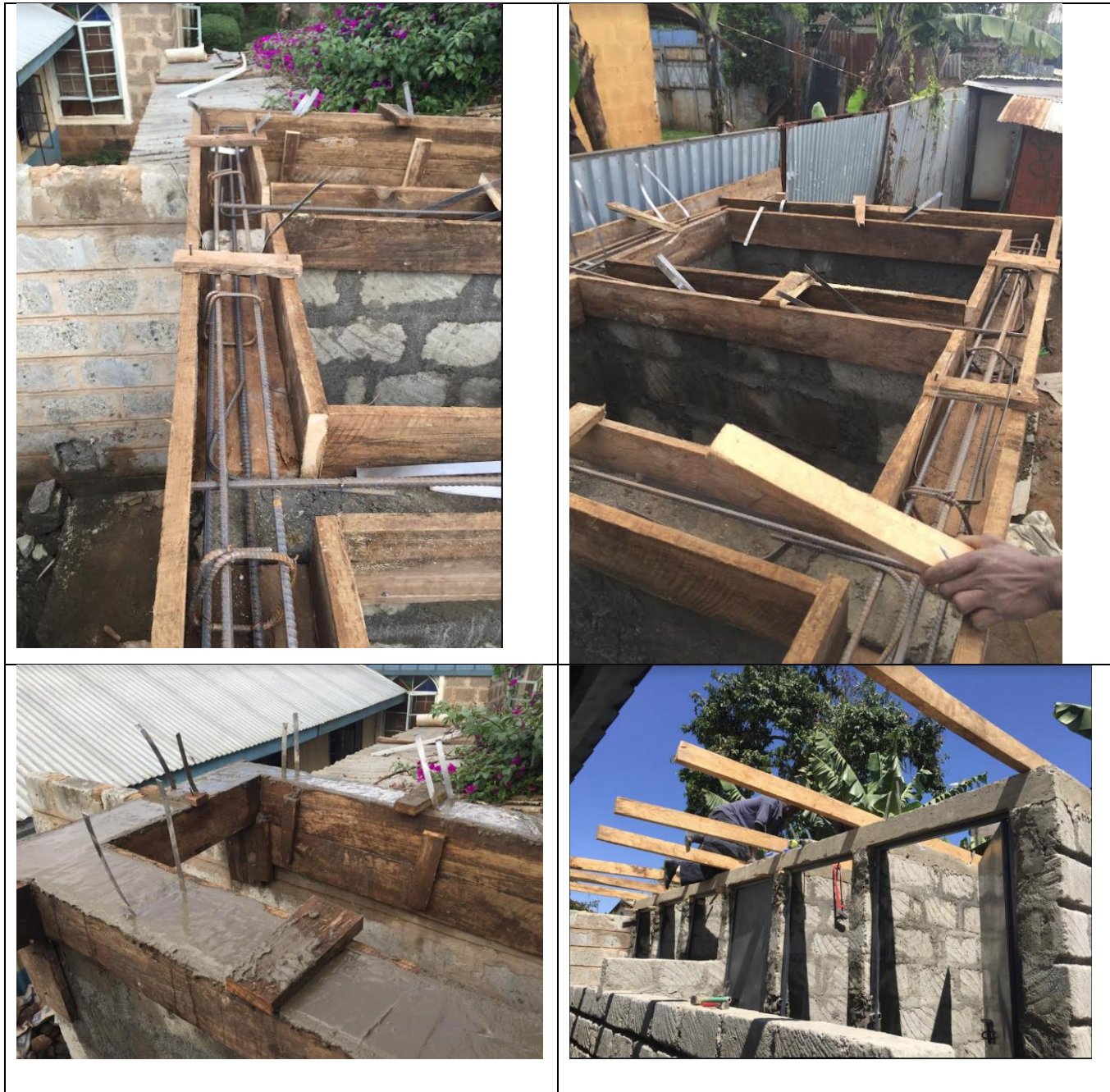
Fig 8: Photos of roof beam structure
